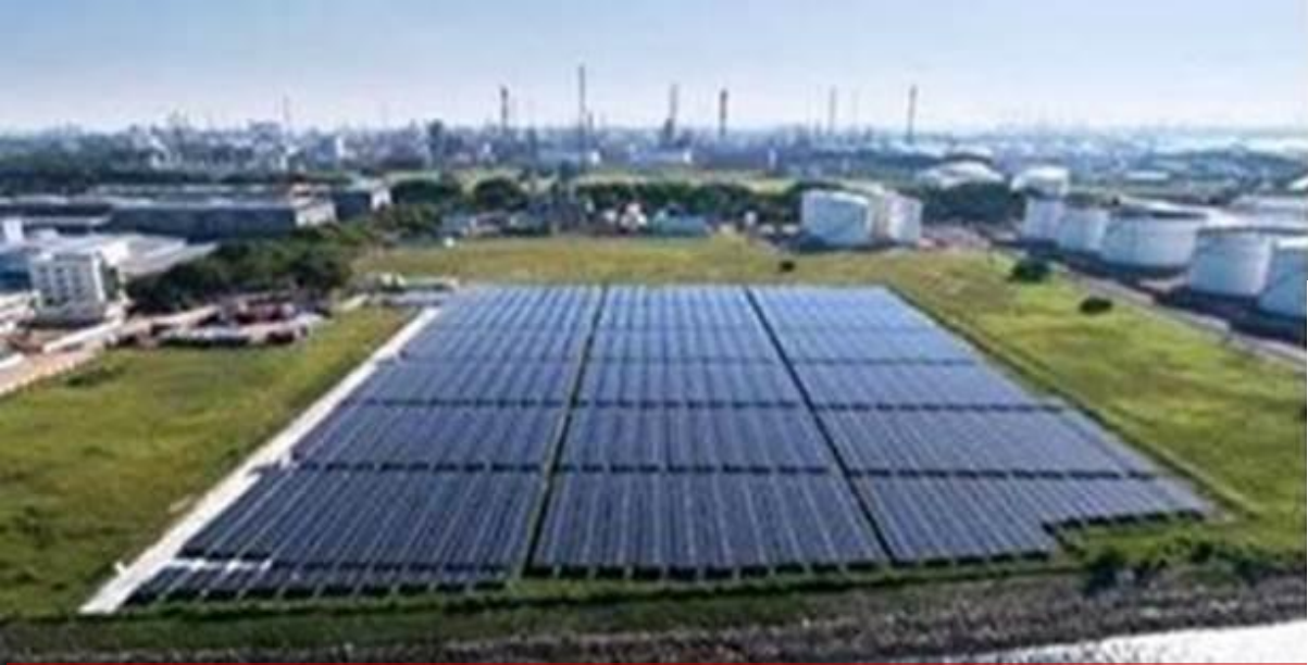
Aerial view of the SolarLand installation on Jurong Island. The system is modular and flexible, allowing JTC to maximise temporary vacant land and redeploy the land when needed. (Credit: JTC)
