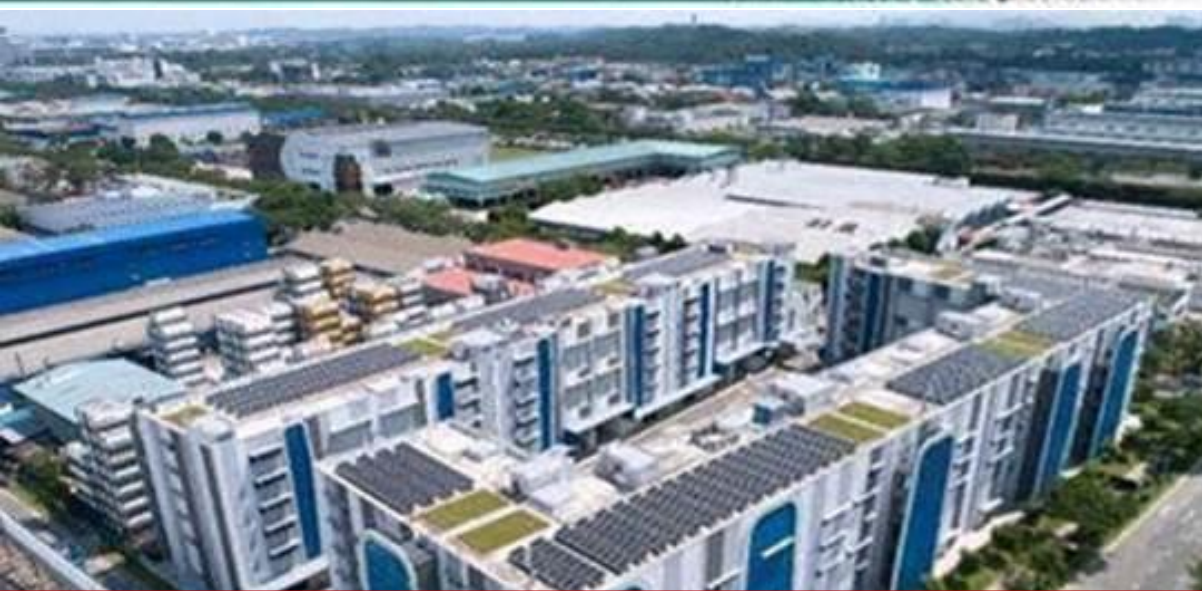
JTC's SolarRoof model at JTC Space @ Gul enables the direct export of solar power generated from industrial rooftops to the national power grid. (Credit: JTC)
