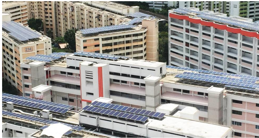
Solar panels on HDB apartment rooftops
