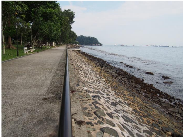
Sloping revetment to prevent coastal erosion
