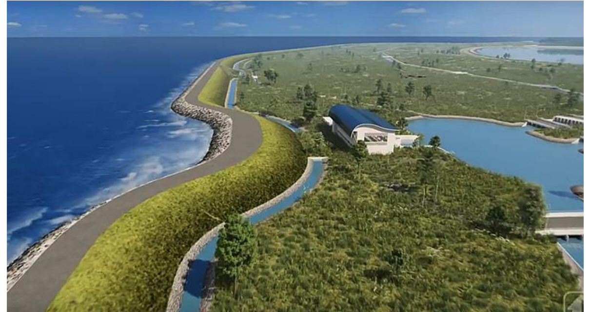
Polder development at Pulau Tekong by Dutch company Royal Boskalis and Japanese company Penta-Ocean Construction
